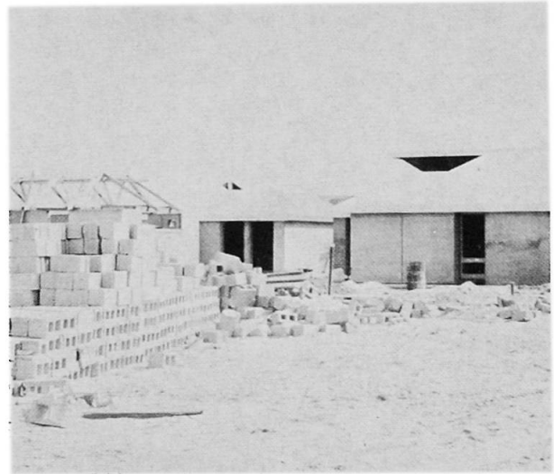
Fig.2: Photograph of typical elevation.
