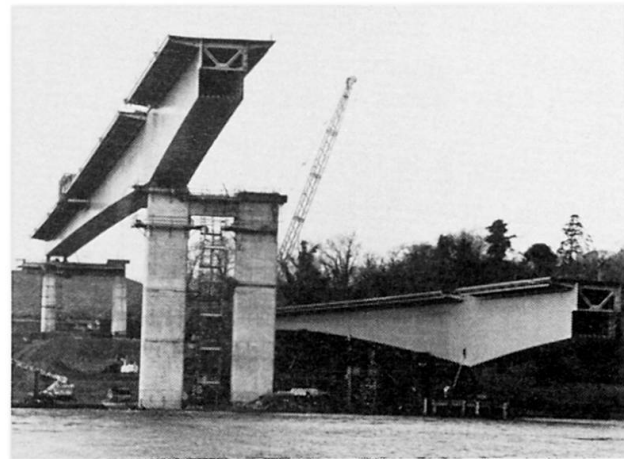
Fig. 9. Sidespan in final position
