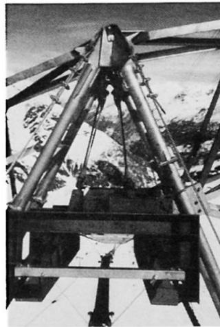
Fig. 6 Head of intermediate pylon
