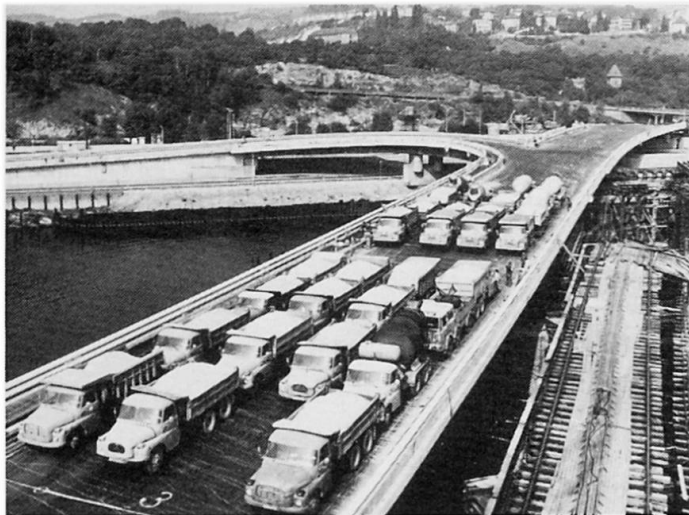
Fig. 10 - Completed half of the bridge under test loading
