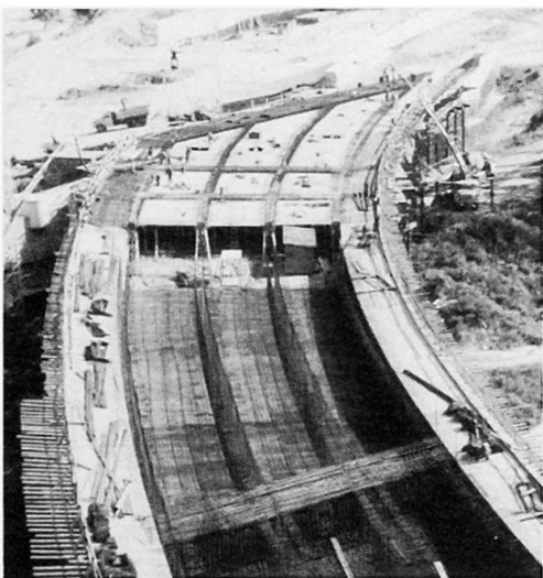
Fig. 9 - Construction phases of the superstructure
