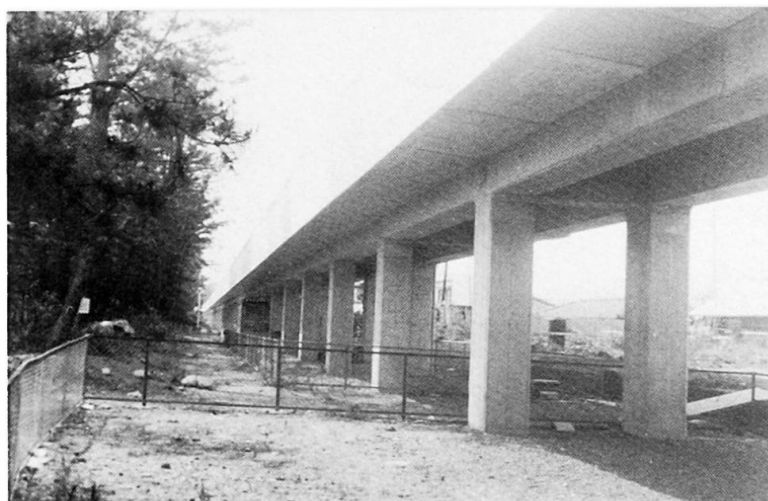
Photo 1. 50-span Concrete Viaduct
