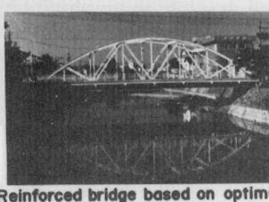
Reinforced bridge based on optimum combination of diagonal hangers.
