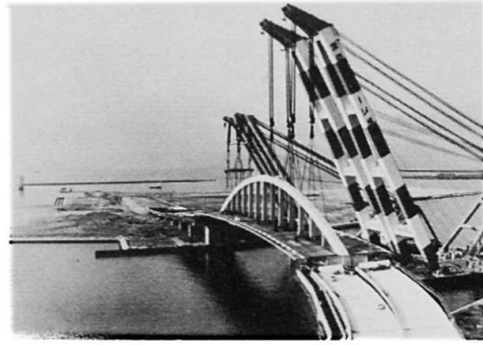
Fig.6 Izumi Otsu Bridge(1976) Span 172.572m, 3000t
