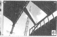
4 Lifting 40 T precast prestressed tied arch girder 30 M span. 5 Tied-arch girders erected and in position 6 6 cm thick folded plate element 12 m. 7 Folded plate elements in position
