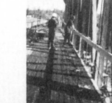
SIOUX NARROWS(1982) Deck Replacement
