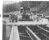
VICTORIA ISLAND Bridge. Deck replacement with prestressed wood panels. Ontario Hydro Ottawa, 1984.
