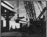
Beams Erected At The Rate Of Six Per Day
