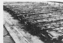
Re-established transverse prestressing
