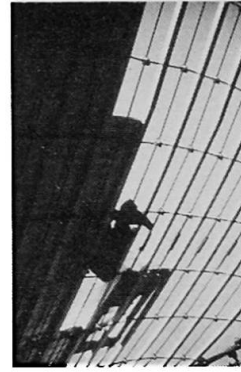
Fig. 17 Vail Town Centre building, USA
