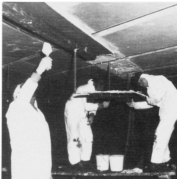
Fig. 3 Bonding of Steel Plates
