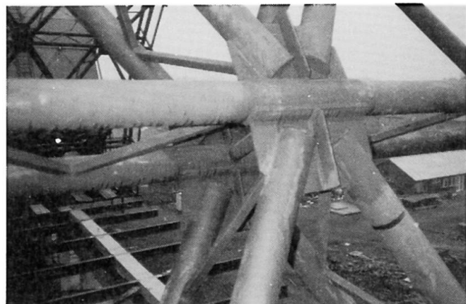
Fig. 3 Special tube-on-tube joint
