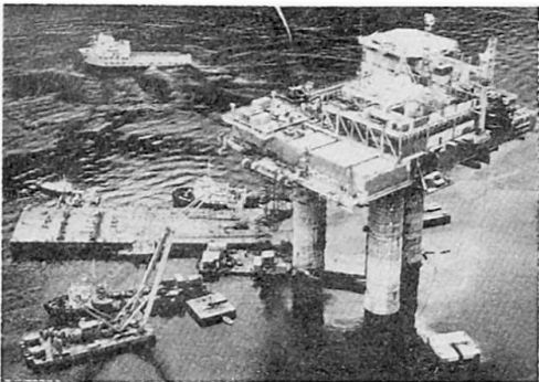
Fig. 3 Platform TCP2, during construction
