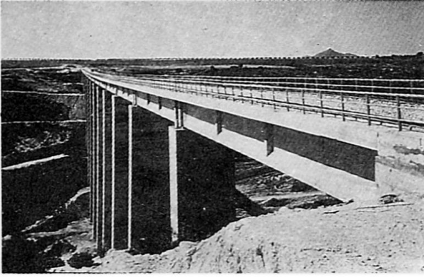
Fig.29 Bridge on Oran-Benisaf line, Algeria
