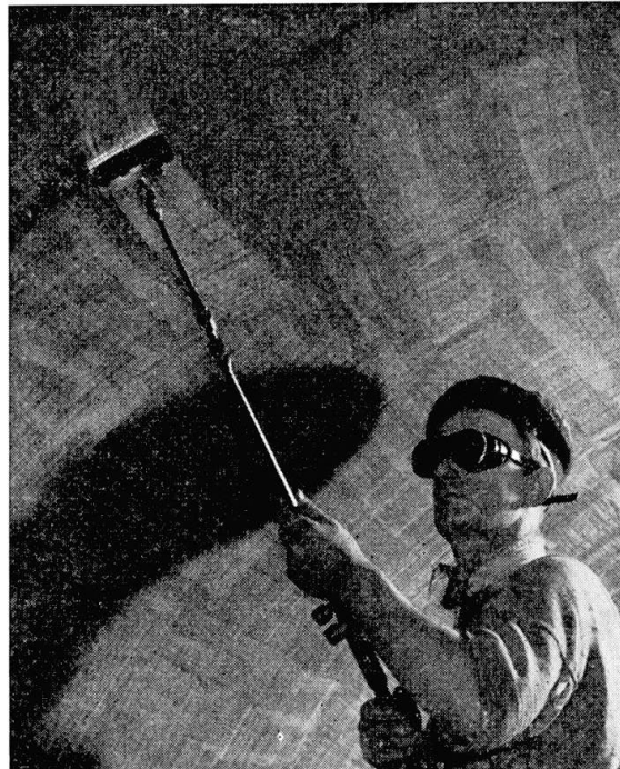
Fig. 12. Flame-cleaning in operation.
