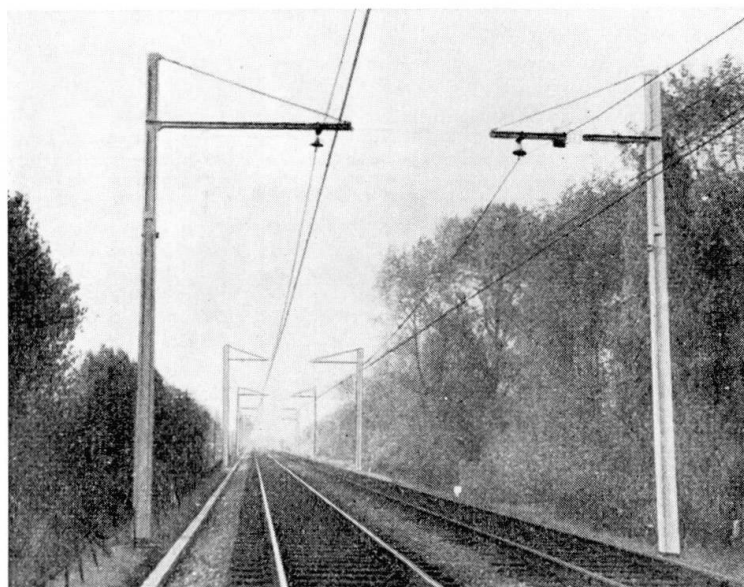
Fig. 1. Prestressed Concrete Cantilever Masts near Southend (England).
