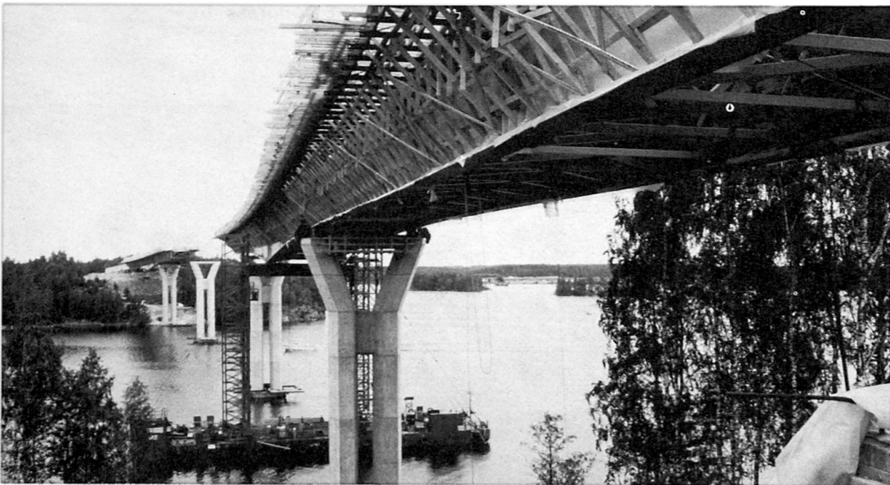
Luukkaansalmi Bridge, Lapeenranta, visited during one of the post Congress tours.
