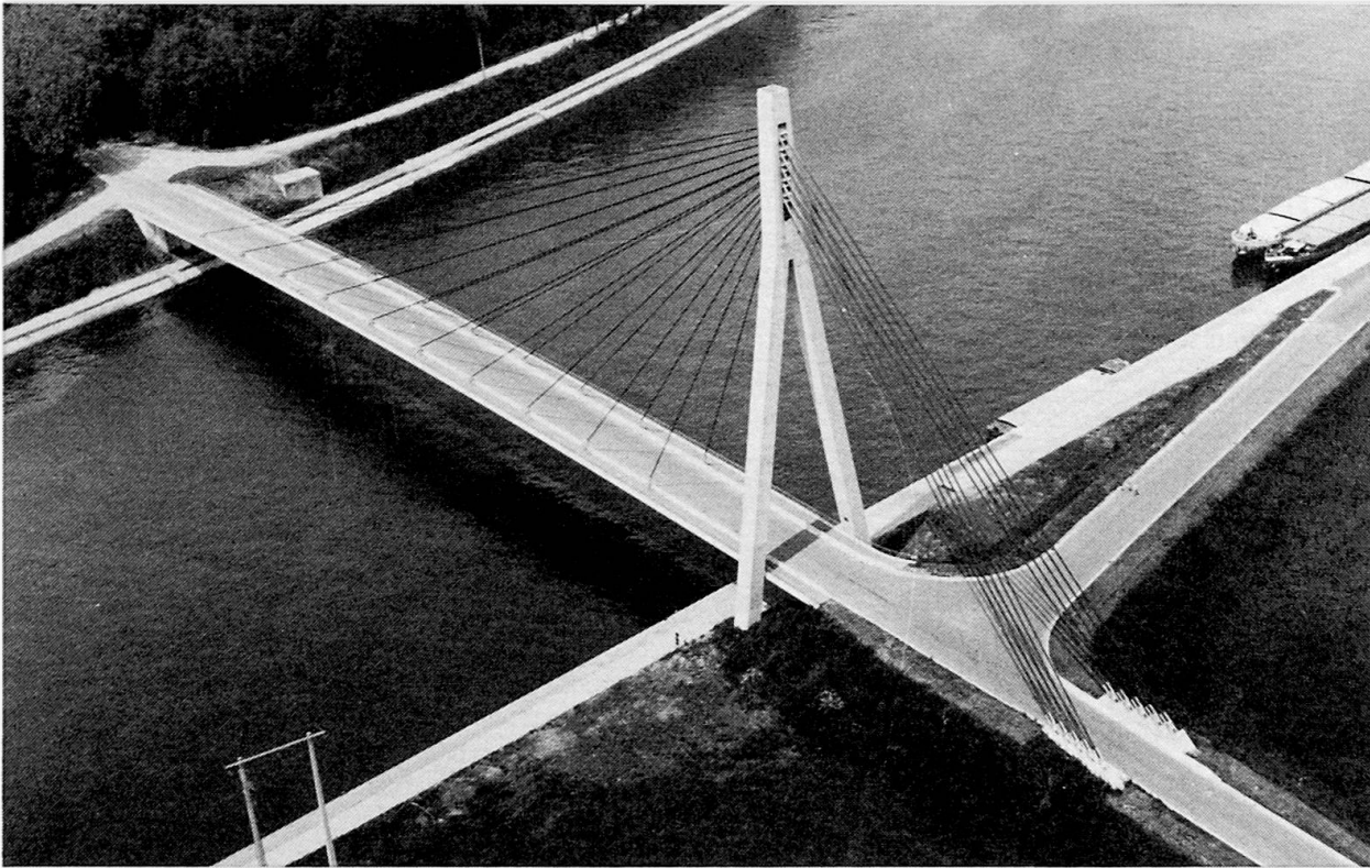
Lanaye Bridge, Belgium (Span 177 m)
