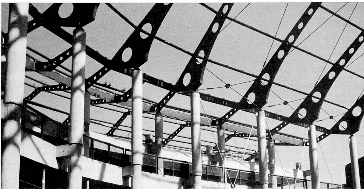
Examples of Industrial, Commercial and Mining Structures
