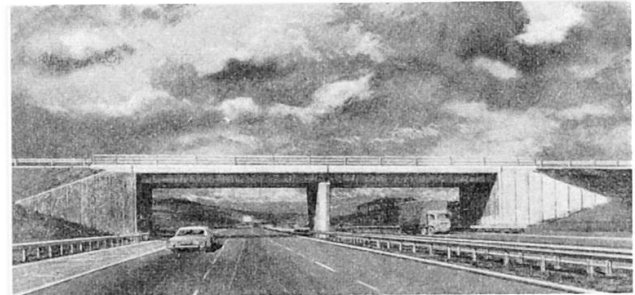
Fig 6 a 2 span overbridge of U beam construction
