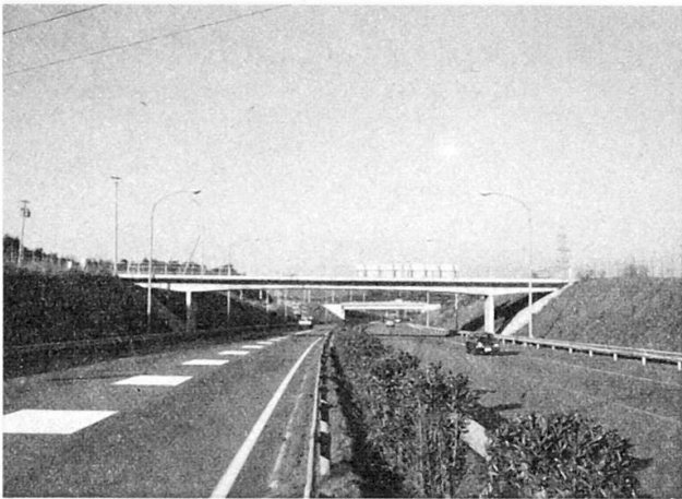
\pi -shaped rigid frame bridge with diagonal members (constructed by Cast in place method)
