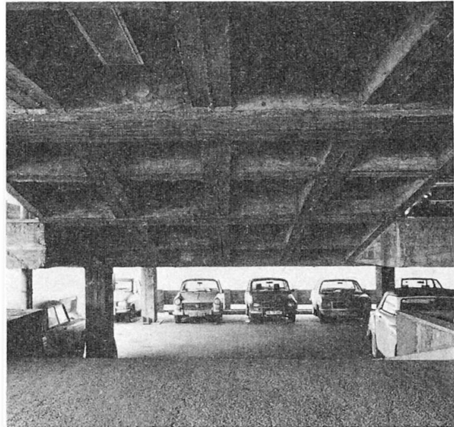
Figure 5. Typical detail from the ramp
