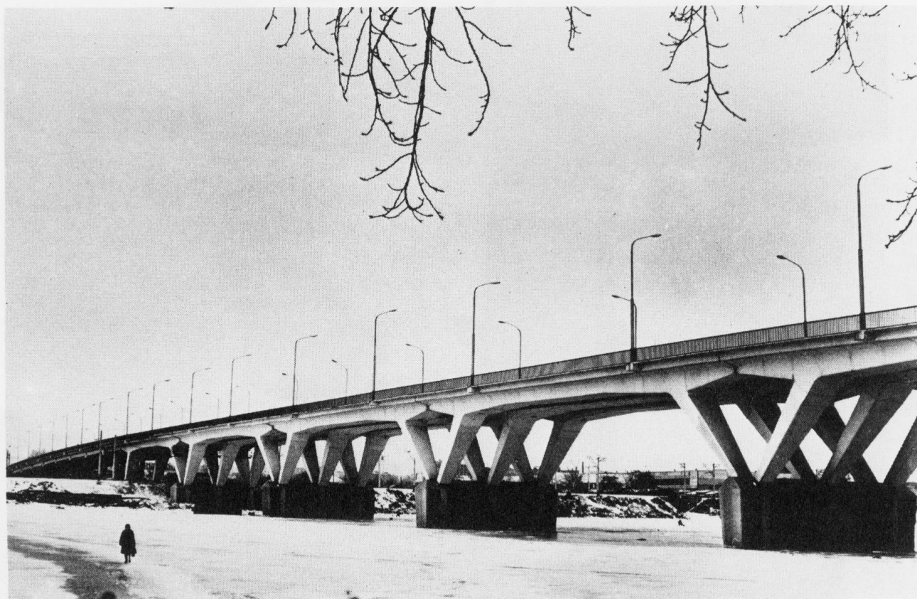
Fig. 1 The general view of the bridge
