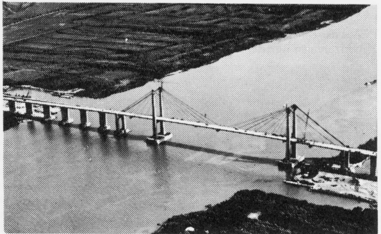
Zárate-Brazo Largo (Argentina) Cable-stayed highway-railway Bridge over Parana River (Techint-Albano)
