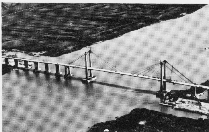
Zárate-Brazo Largo (Argentina) Cable-stayed highway-railway Bridge over Parana River (Techint-Albano)
