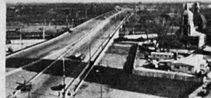
Rizhskaya Flyover in Moscow Concrete spans from 25 to 33 m Composite steel continuous girder with spans from 32 to 44 m
