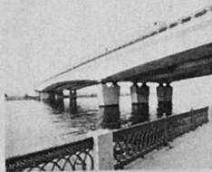
Bridge over the River Moscow Concrete continuous girder with spans 62 \cdot 114 \cdot 62 m (for combined traffic of city vehicles and Metro trains)
