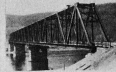
Steel Railway Bridge on the Baikal-Amour Railway Line Steel continuous girder with spans 110 \cdot 132 \cdot 110 m
