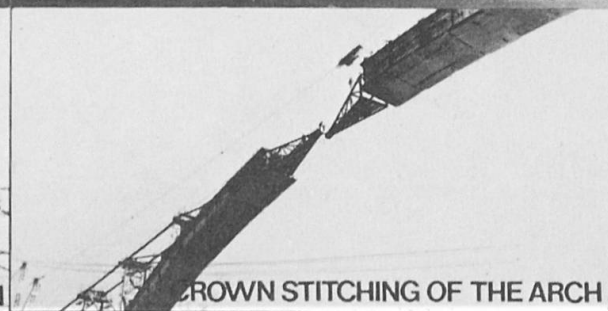
CANTILEVER METHOD OF CONSTRUCTION OF THE BRIDGE ARCHES
