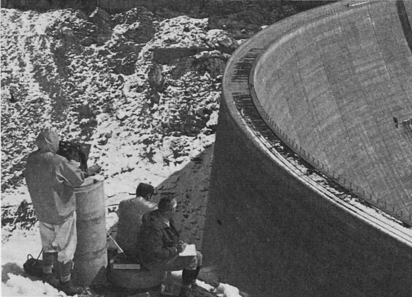
The Mekometer used for dam control measurements
