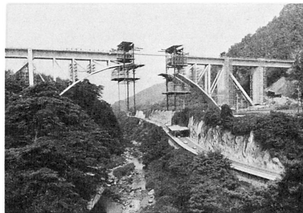
Photo 5 Akayagawa Bridge under construction
