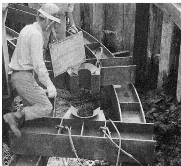
Photo 2 Guiding ring beams for pipe-pile-wall foundation
