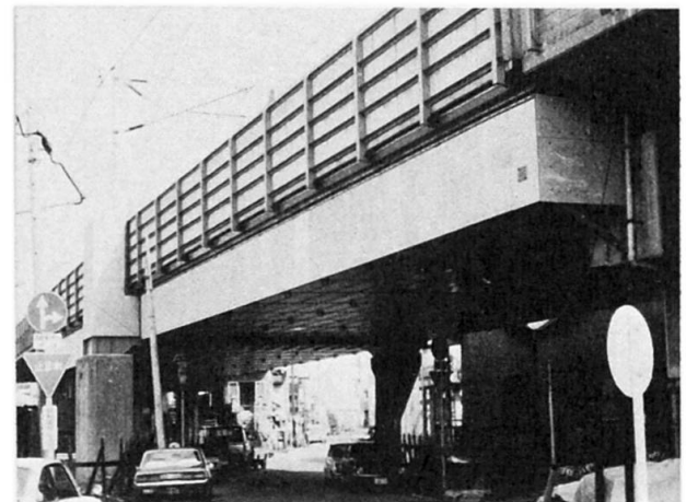
Photo 2 Bridge after improvement
