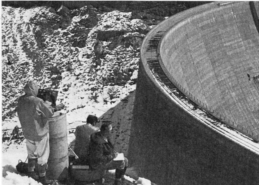
The Mekometer used for dam control measurements
