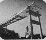
Sennett (single bridge) 3 spans: 51 + 62 + 71 + 63 + 8 + 50 + 36 = 354 m steel weight: 1,220 t recast concrete slab: 13,890 m 3
