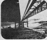
Bergbach (twin bridge) 6 spans: 70 + 4,775 + 60 = 440 m steel weight: 1,166 t precast concrete slab: 11,620 m 3
