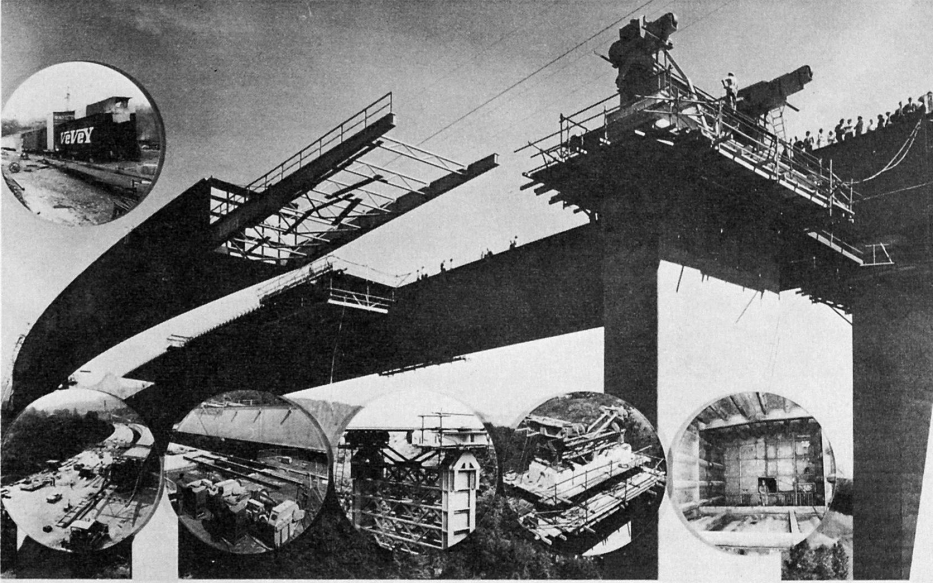
Sennett (single bridge) 3 spans: 51 + 62 + 71 + 63 + 8 + 50 + 36 = 354 m steel weight: 1,220 t recast concrete slab: 13,890 m 3
