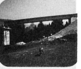
Louvauch (single bridge) 4 spans: 52 + 65 + 52 + 52 = 221 m steel weight: 260 t cast in place concrete slab: 2,260 m 3
