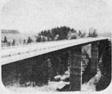
Gilwe (twin bridge) 3 spans: 56 + 71 + 56 = 183 m steel weight: 520 t precast concrete slab: 4,100 m 3
