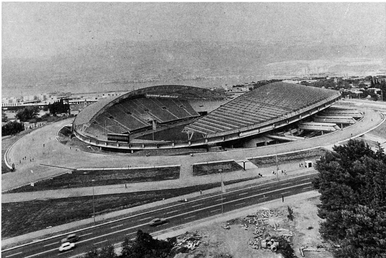
Fig. 1 View to the City Stadium
