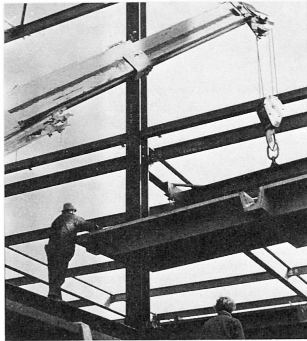
Precast floor units being lowered onto steel frame
