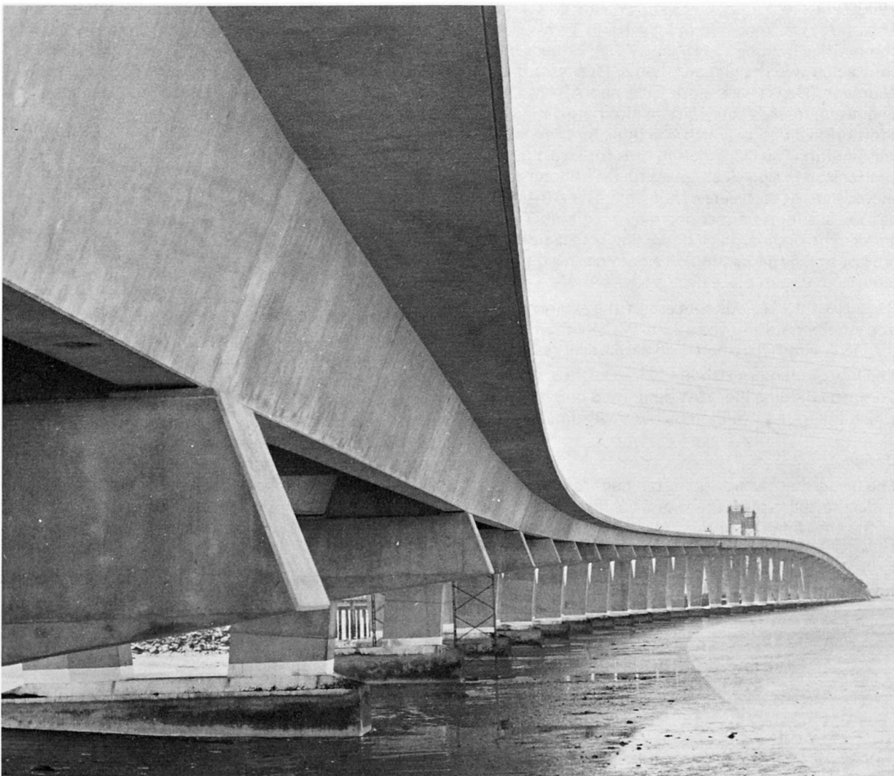
Fig. 4 Prestressed lightweight concrete girders
