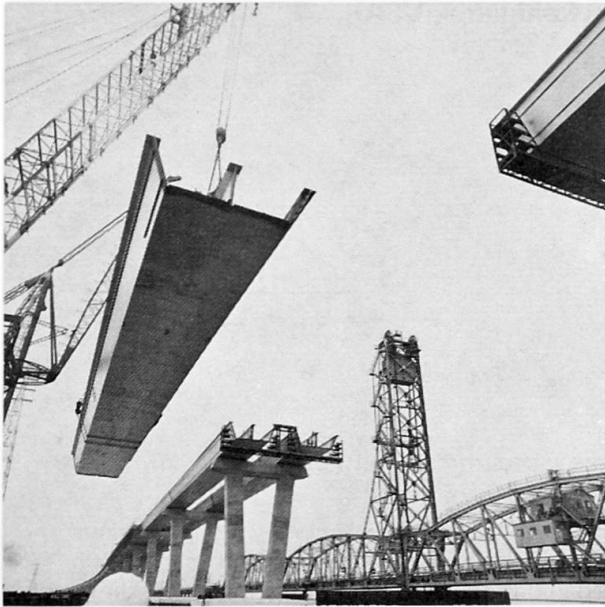
Fig. 2 Lifting of a trapezoidal steel box girder
