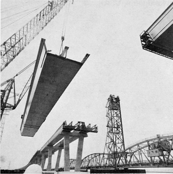
Fig. 2 Lifting of a trapezoidal steel box girder
