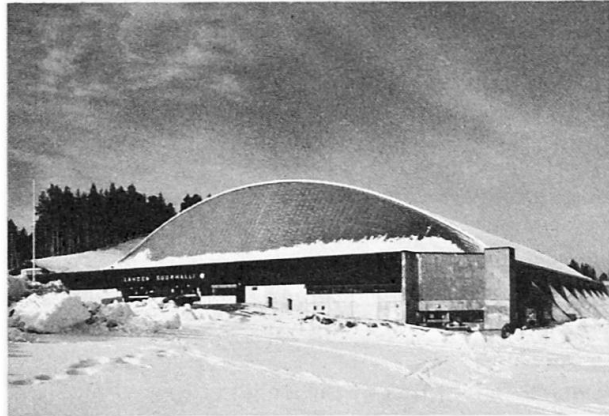
Facade, from the south side
