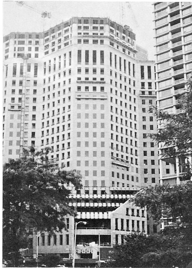
Fig. 4 One Magnificent Mile building under construction
