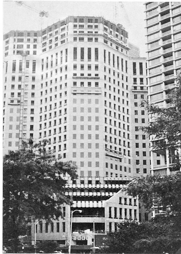
Fig. 4 One Magnificent Mile building under construction
