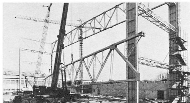
Fig. 2 Erection of steel trusses
