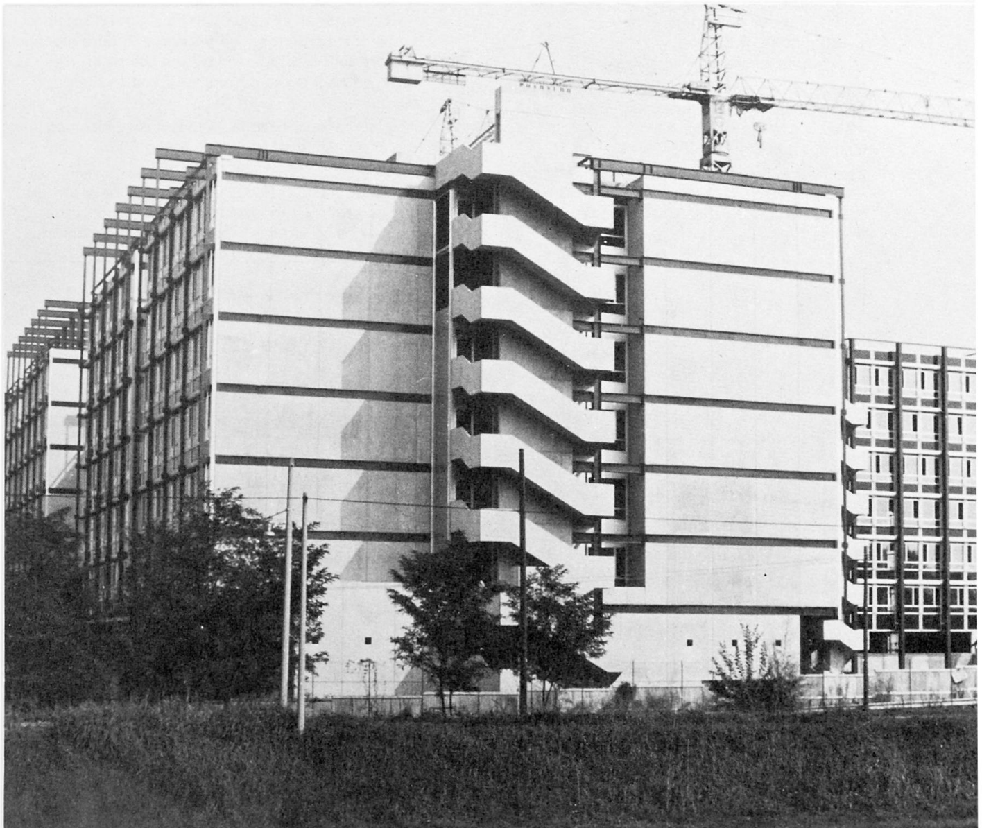
Fig. 2 The building in the final stages of construction
