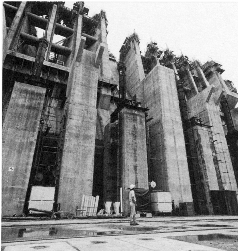
Hollow gravity dam
