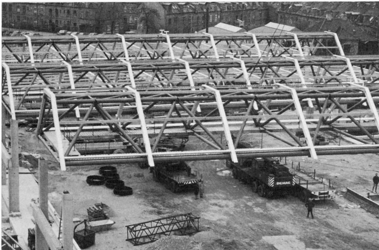
Building under construction
