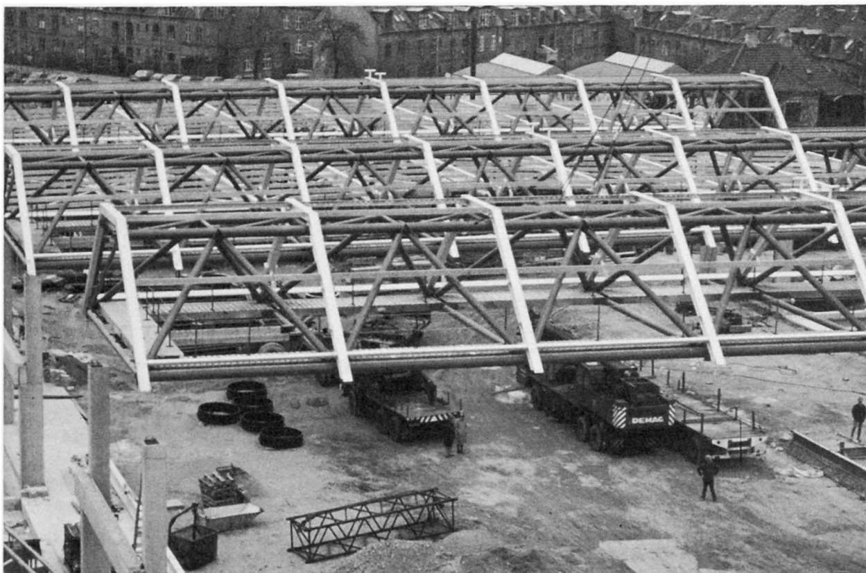
Building under construction
