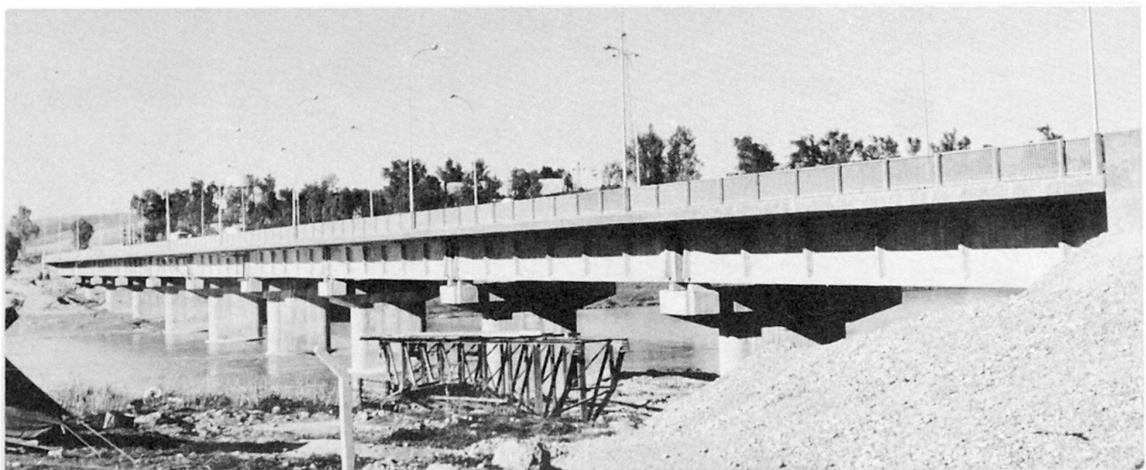
View of the completed bridge
