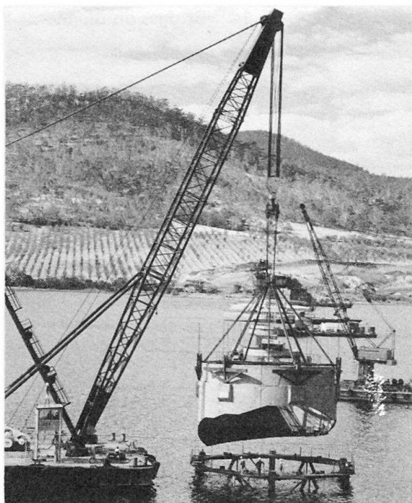
Fig. 4 Lowering first segment Pier 2 Cofferdam
