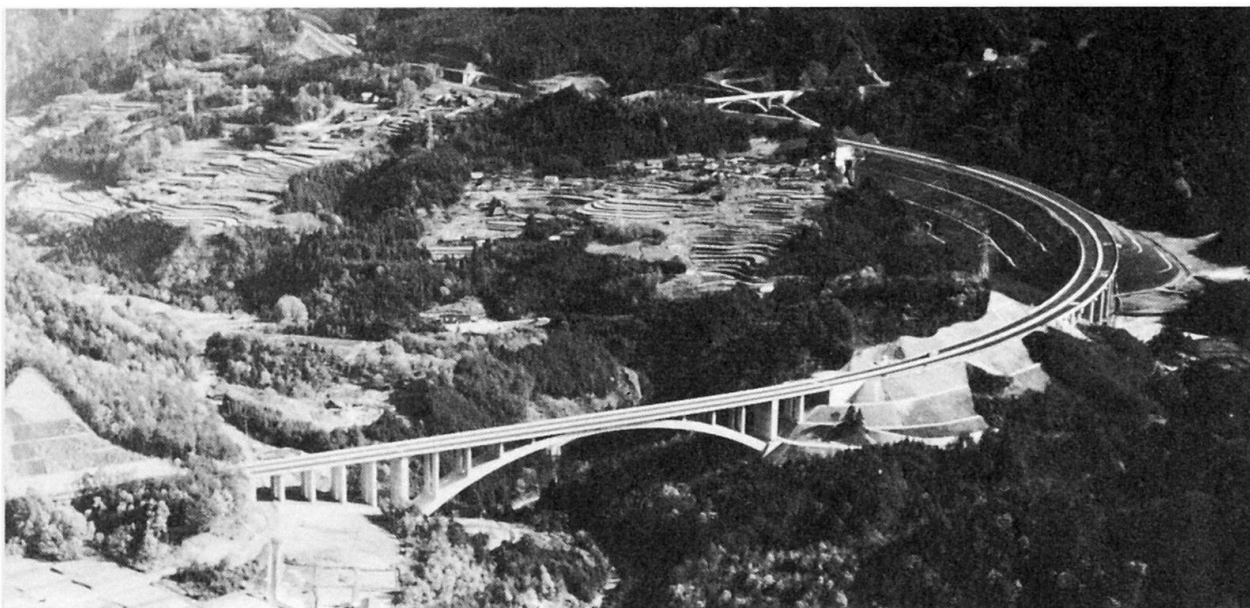
Fig. 4 View of the bridge completed
