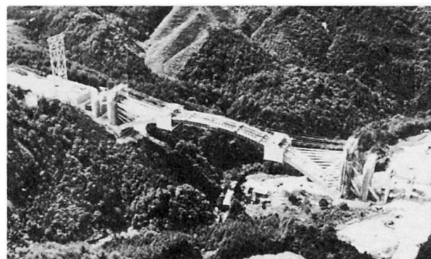
Fig. 2 Construction over a steel girder arch
