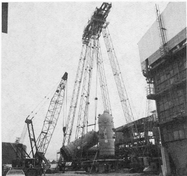
Fig. 4 Lifting frame during the erection of 2 reactors with a weight of 250 t each, in Malaysia
