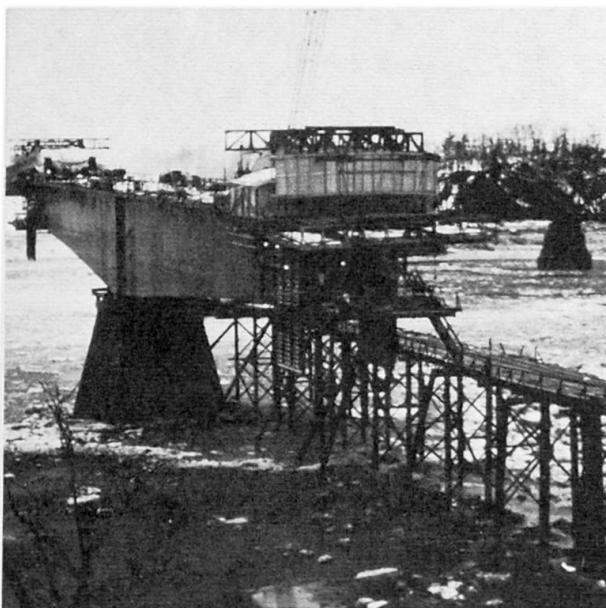
Fig. 1 East span advancing under winter conditions
