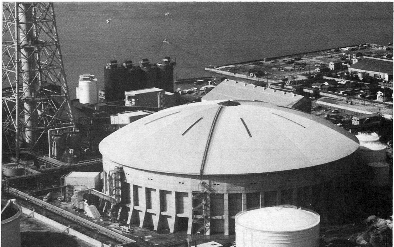
View of the storage coal structure
