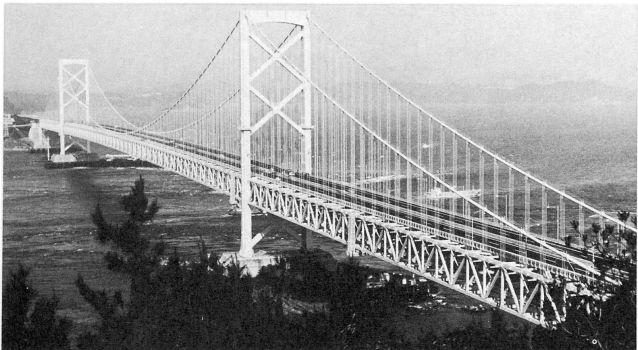
View of the Ohnaruto Bridge
